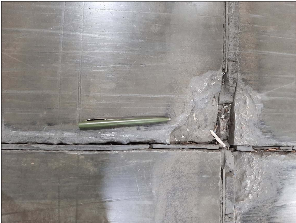
Photo 4: Photo of a crack along a concrete seam at A349.
