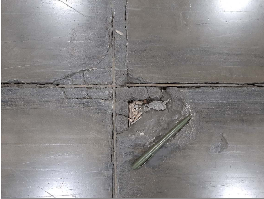
Photo 3: Photo of a crack along a concrete seam at A335.
