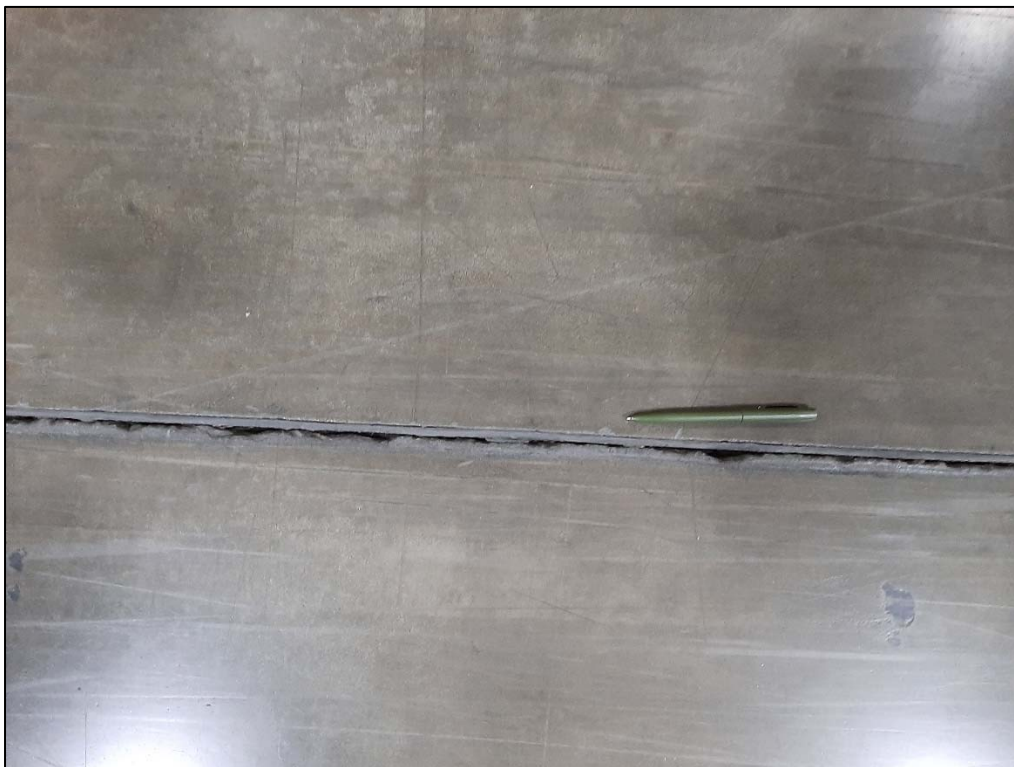
Photo 2: Photo of a gap in the caulk along a concrete seam near location A249.
