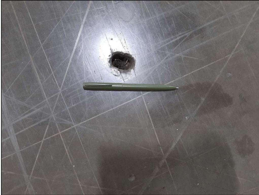
Photo 1: Photo of small hole in concrete floor near Door 1.
